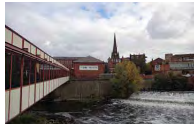
Fig. 5.5.4 Above: Carpark on Forge Island
