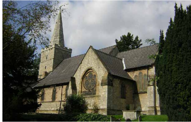
Fig. 5.2.1: Grade II* listed St Bartholomews Church.
