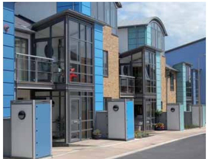
If frontage storage is the only option it should be well integrated into the building design
