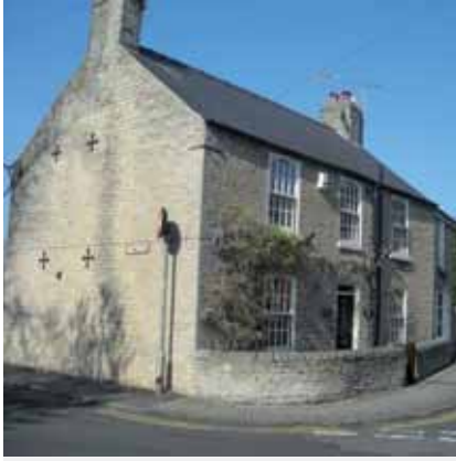
Double pitched roofs with gable ends like this one in Tickhill, Doncaster, are one of the predominant roof forms in South Yorkshire
