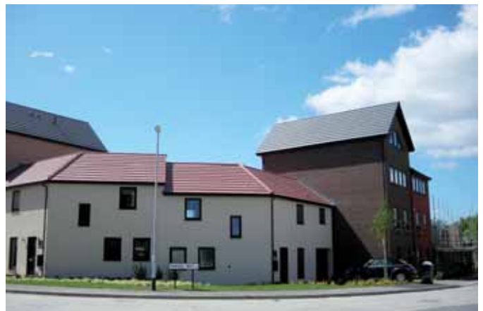
A new corner type that fails to make the most of the corner, leaving the main face of the corner too low, blank and inactive
