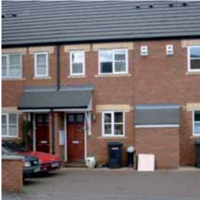
Standard, small terraced house types do not perform well in meeting Code for Sustainable Homes standards, in particular for storage of waste and recycling and access to rear gardens
