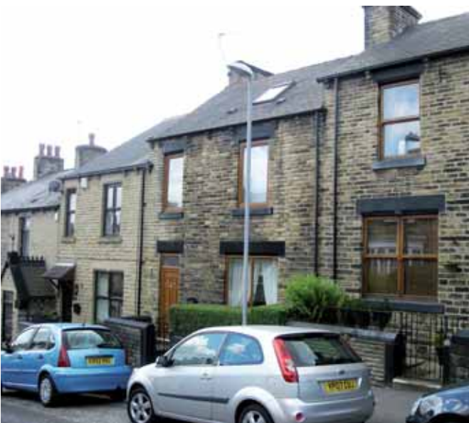
The stepped arrangement, as here in Old Town, Barnsley, means the roof line follows the slope of the ground for a better roofscape
