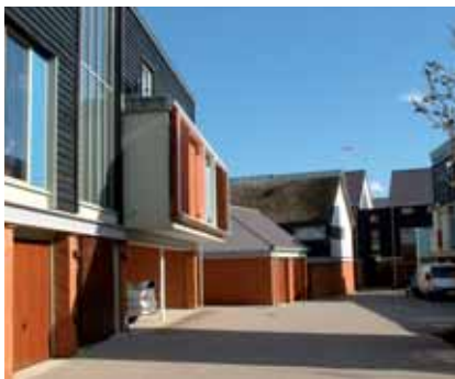
A level surface shared space in a mews
