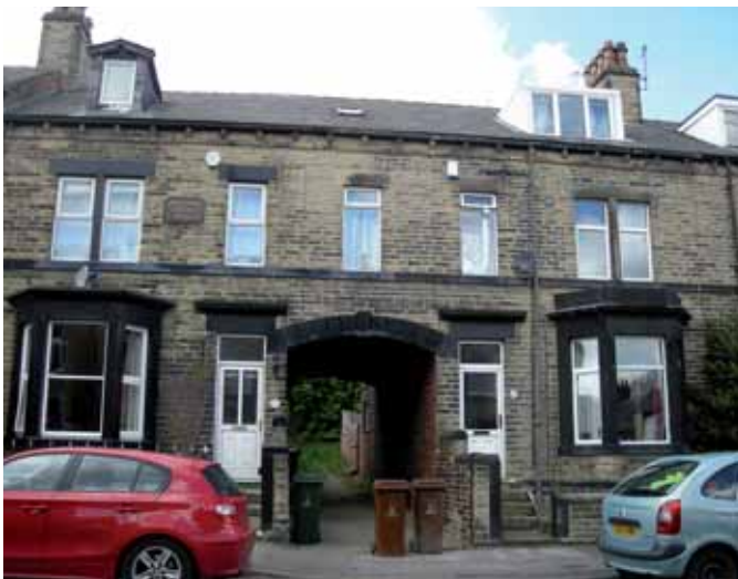
The traditional 'ginnel' is a robust and adaptable feature that allows for access to waste and recycling storage that remains out of view
