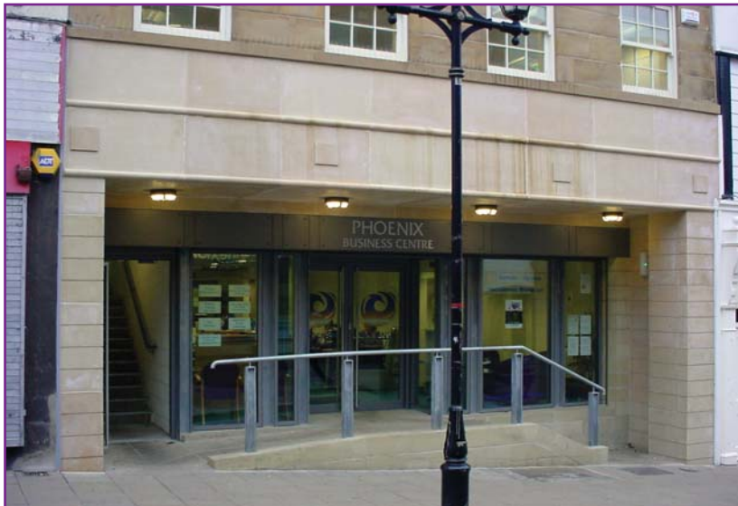
New ramp and steps create a fully accessible entrance set back from the street frontage
