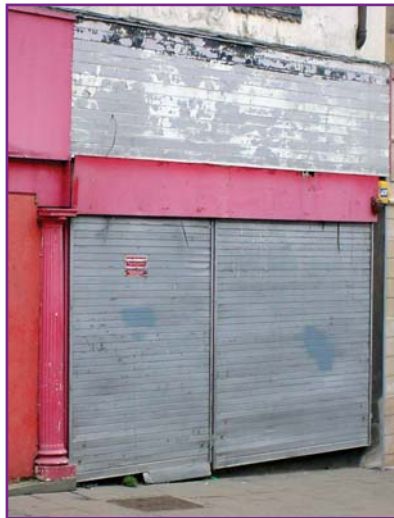
Unacceptable exterior solid shutter
