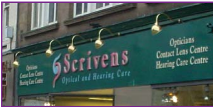
A traditional example of fascia illumination
