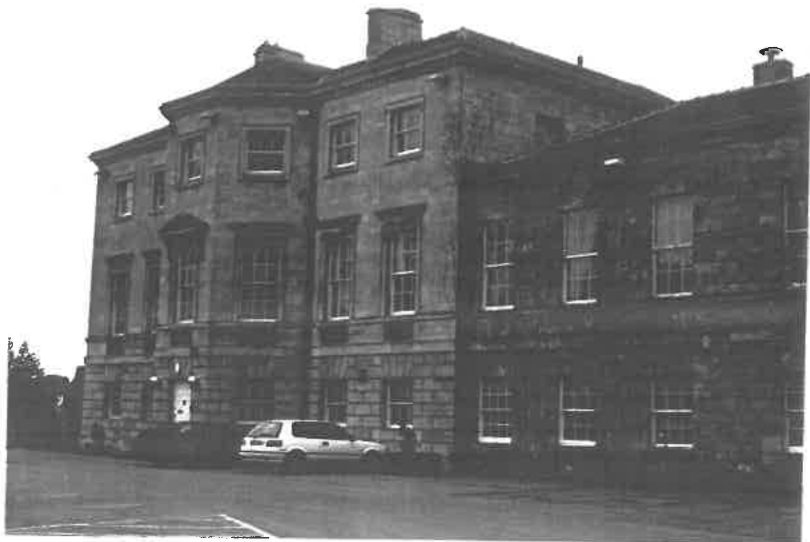
9 Aston Hall: from north-west, 1996
