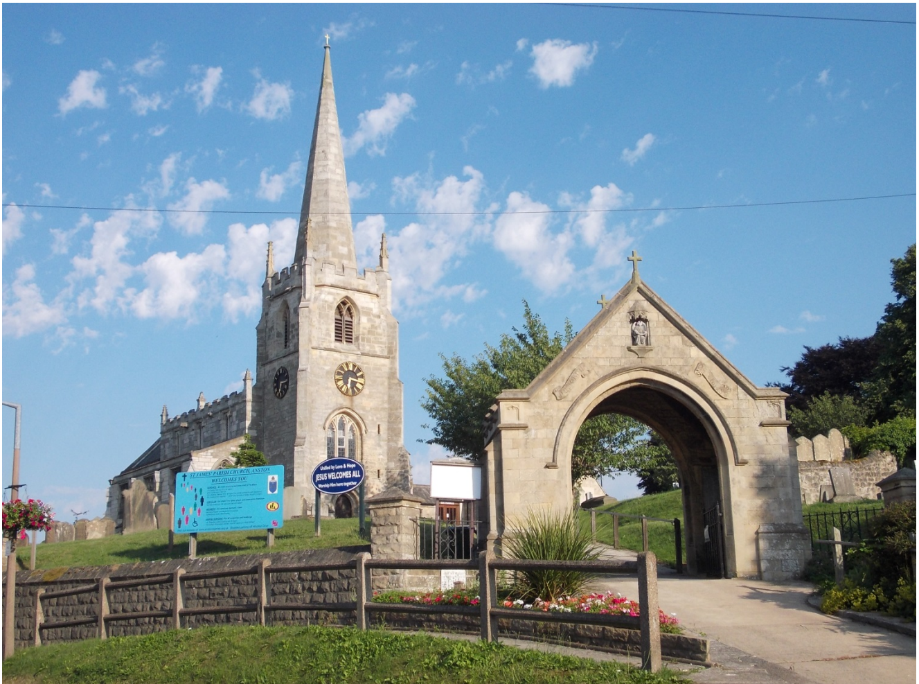
Figure 3 The western elevation with tower and lych gate taken from the junction of Sheffield Road and High Street
