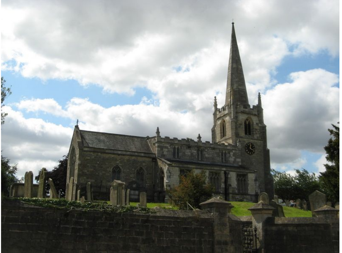
Figure 4 Church of St James, north elevation, taken from Sheffield Road
