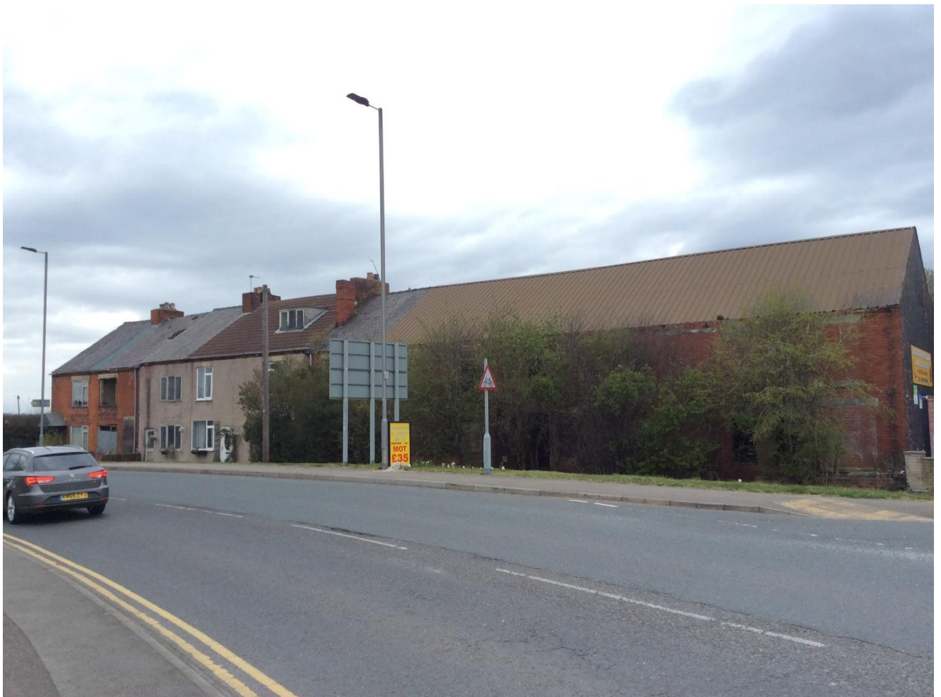
Derelict building formerly in business use
