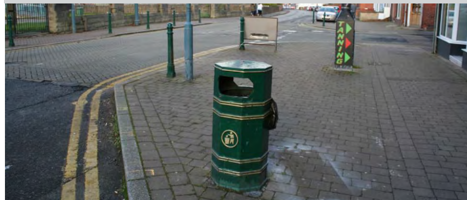
Figure 3.9 Lack of maintenance and poor quality materials
