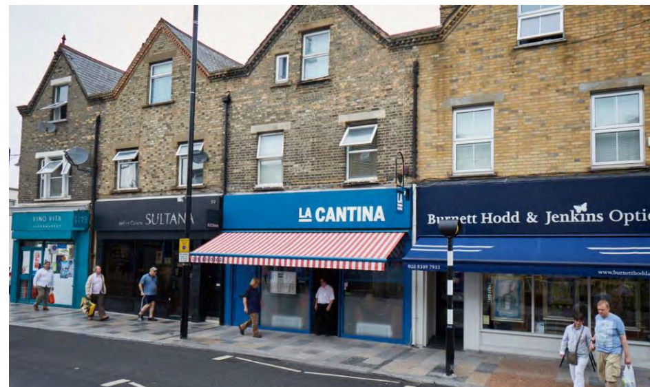
Figure 4.21 Example - Unified shop fronts and high quality materials, Eastgate Street, Sidcup
