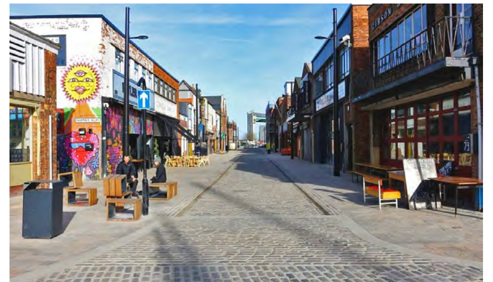
Figure 4.14 Example - Improved shop fronts and shared surface, Humber Street, Hull
