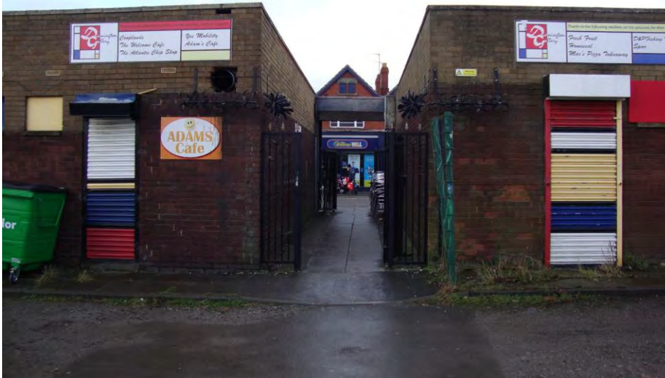
Figure 3.2 The market gateway to Laughton Road is unappealing
