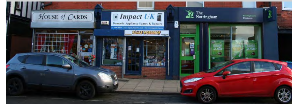
Figure 3.12 Modern shop fronts detract from the character of buildings on Laughton Road
