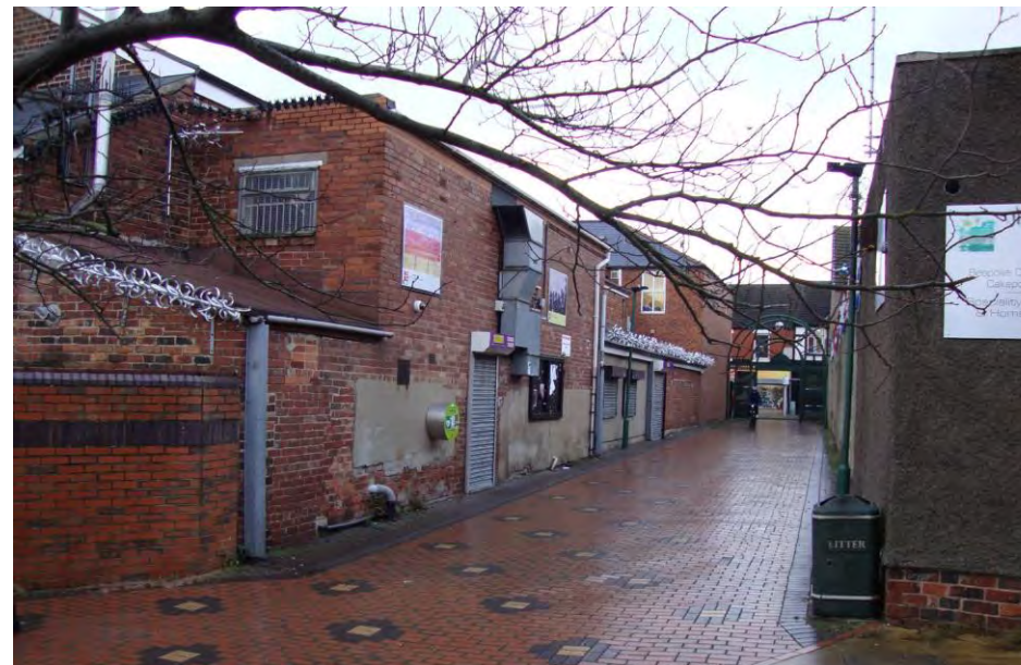
Figure 3.1 Materials detract from the gateway between Constable Lane and Laughton Road
